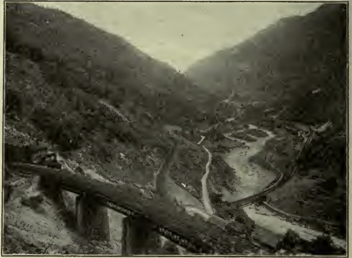
FIG. 556. — The St. Gothard Railway on the south side of the Alps. Here are three tracks one above the other, for the railway enters the mountain and swings around in two great circles, coming out each time at a higher level.
